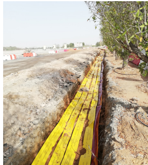
Figure K.77 Typical cable route marker (DEWA)
