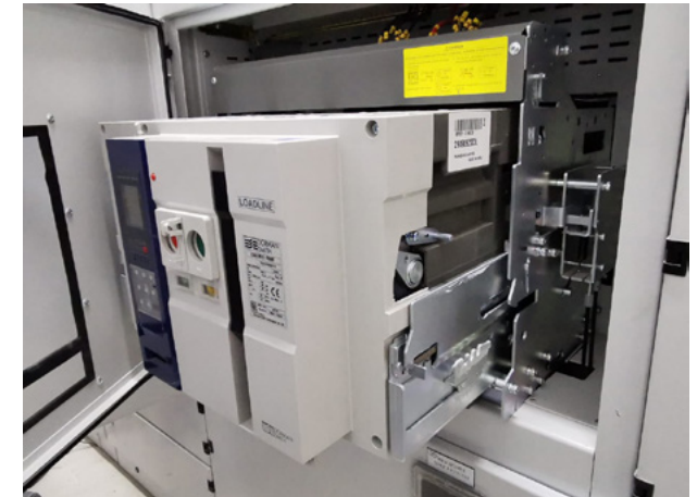
Figure G.2 Typical fully withdrawable four-pole circuit breaker
