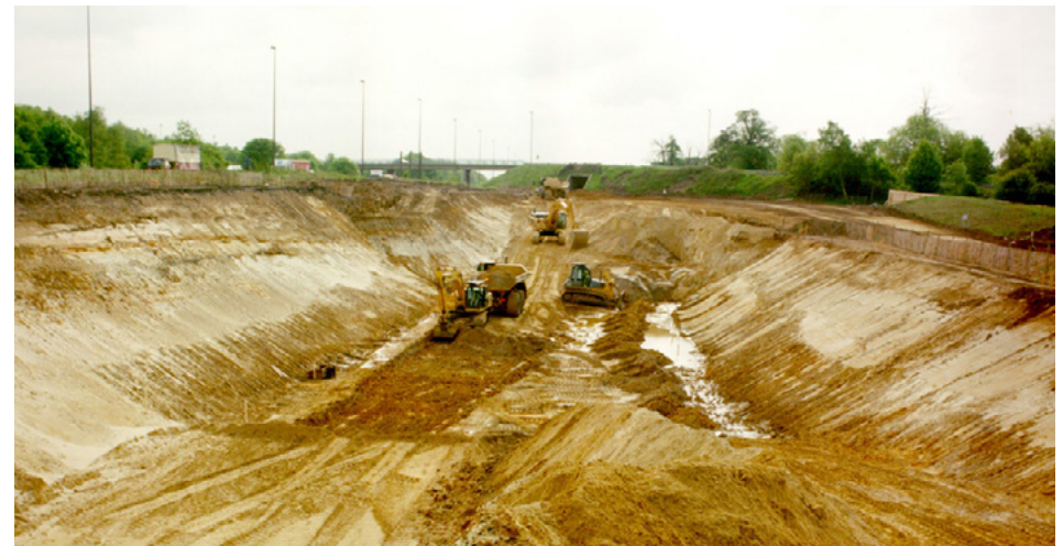
Figure K.60 Open cut excavation
