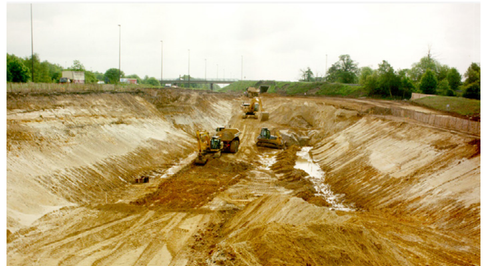
Figure F.22 Open cut excavation
