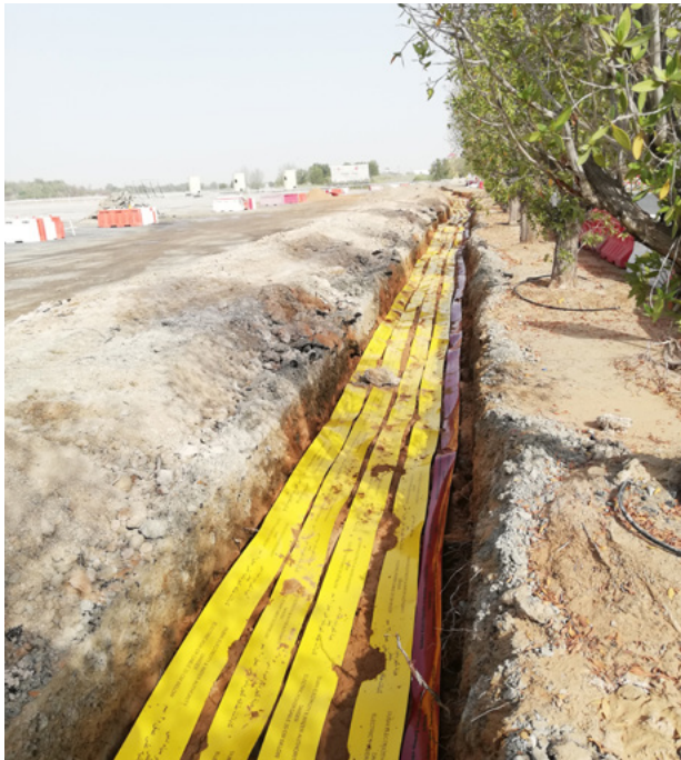
Figure G.22 Typical cable route marker (DEWA)
