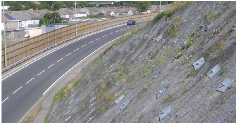
Figure K.62 Installation of soil nailing system
