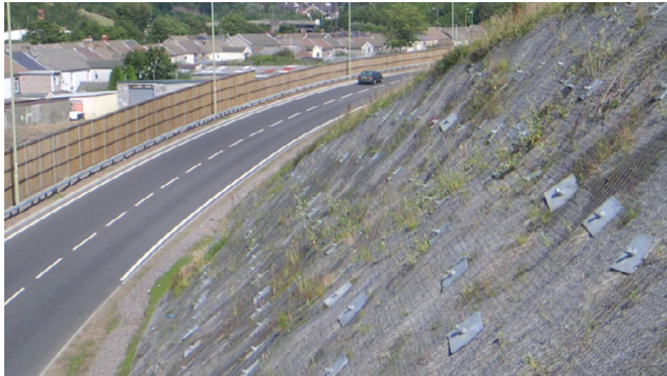
Figure F.24 Installation of soil nailing system
